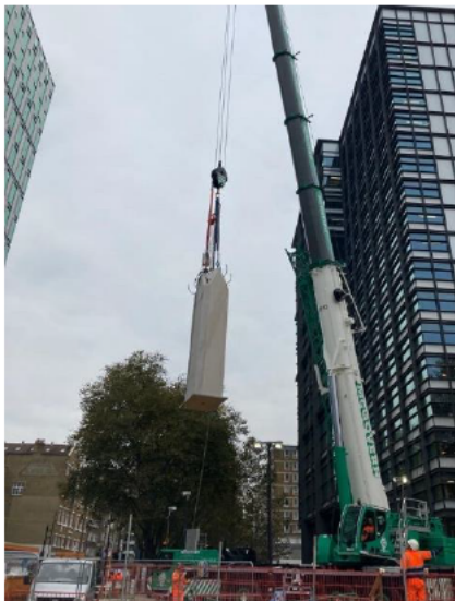
Superstructure pre-cast concrete column crane lift
